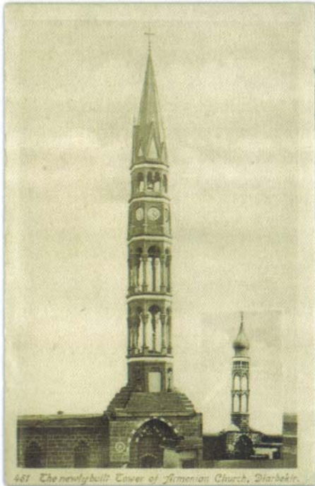
461 The newly built Tower of Armenian Church, Diarbekir.
