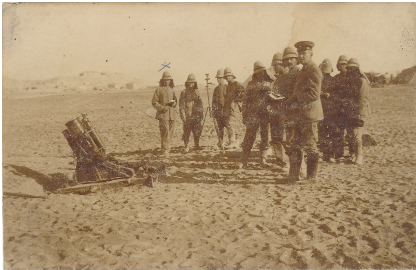
Fig. 1: Pioneers of Minenwerfer-Abteilung 351 (Mine Thrower Section 351) in front of their 7.58 cm light mine thrower in the desert of the Sinai Peninsula. The operator crew consisted of 5 to 6 men. The thrower was loaded via the muzzle, the range was 1050 m, the projectile rate was 6 shots per minute, the projectile weight was 4.6 kg and was effective through fragments. 3
